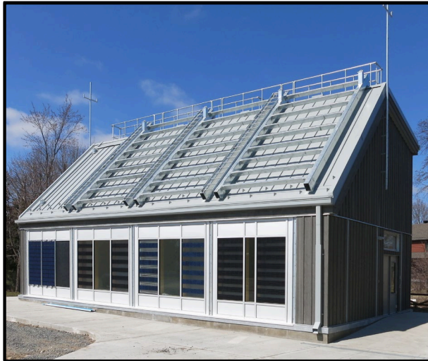
Future Buildings Laboratory
