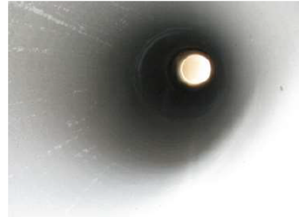
Fig 1. 750mmØ precast pipe (1 of 3)
