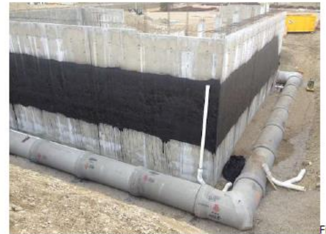
1. 750mmØ precast pipe (1 of 3)
