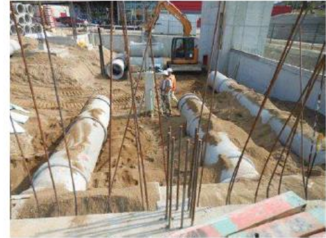
Fig 3. Pipes in trench prior to backfill
